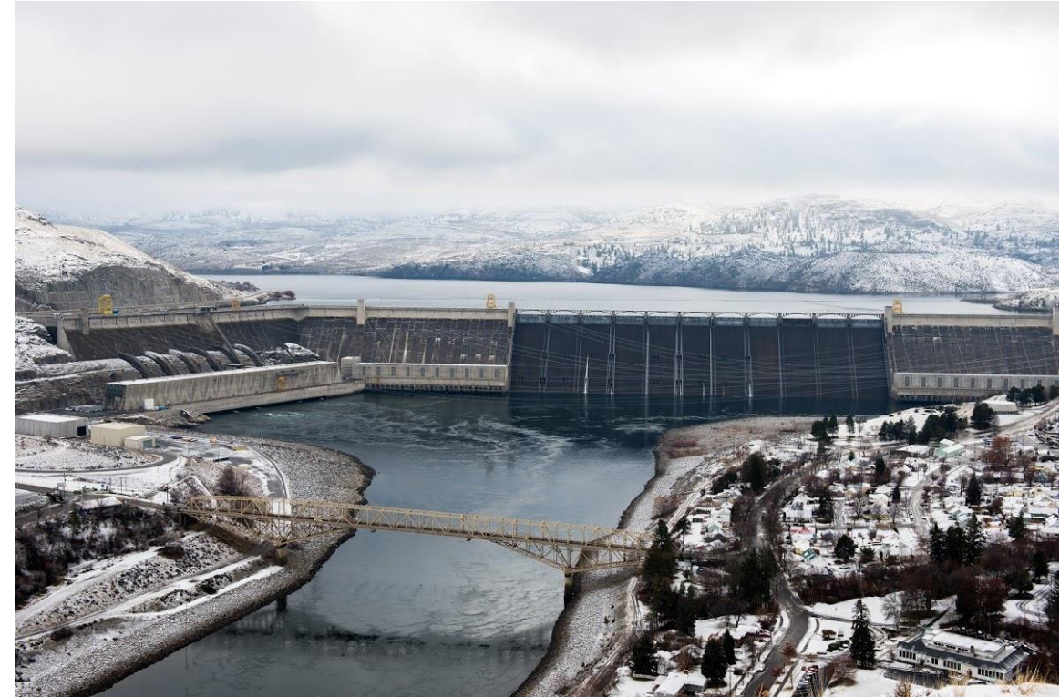
The Grand Coulee Dam in the winter. Courtesy of the Bureau of Reclamation.
