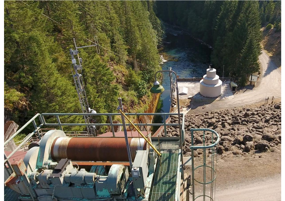
EWEB's Trail Bridge dam and powerhouse on the McKenzie River.
