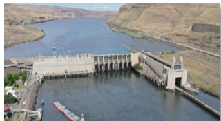
Lower Monumental 6 Units 930 MW*
