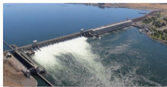
McNary 14 Units 1,120 MW*
