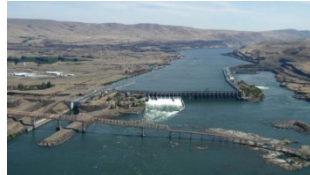
The Dalles 22 Units 2,080 MW*
