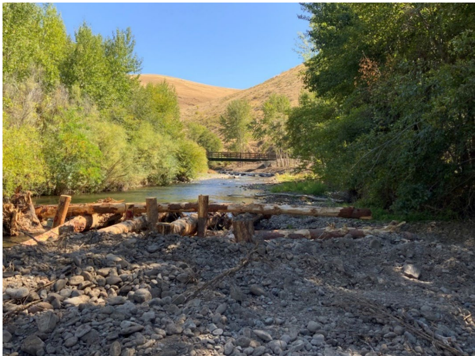
Figure 1: 2023004(Tucannon PA-26) LW Structure1
