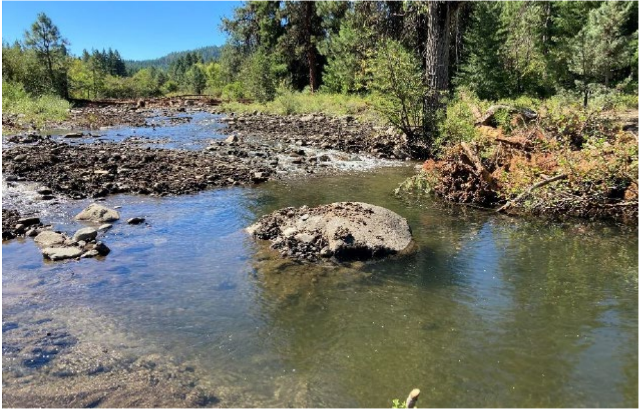
Figure 27: 2023072: Leave pool, rock and margin deflector jam
