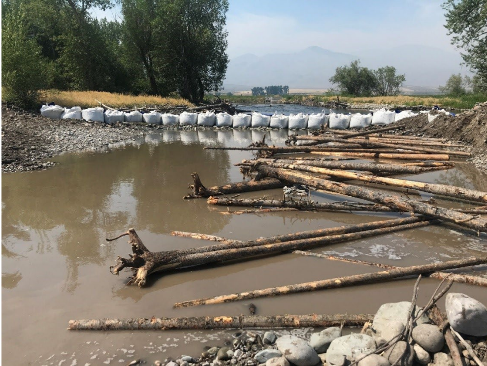
Figure 21: 2023070(Eagle Valley)Coffer Dam
