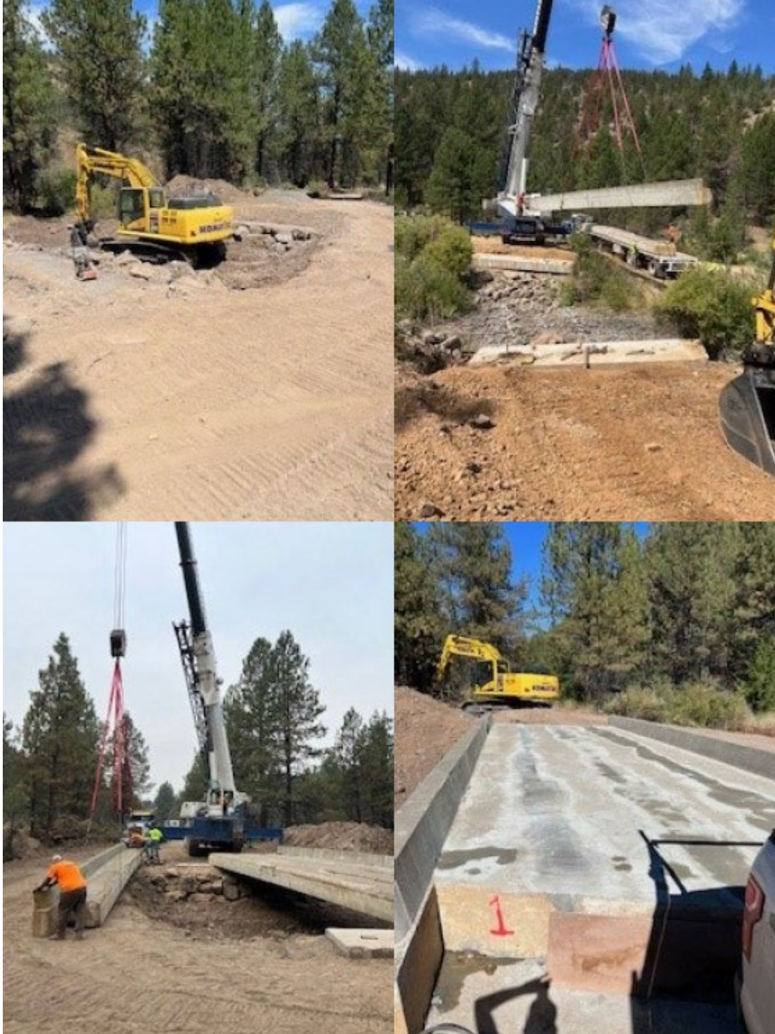
Figure 25: 2023071: Culvert removal and bridge placement
