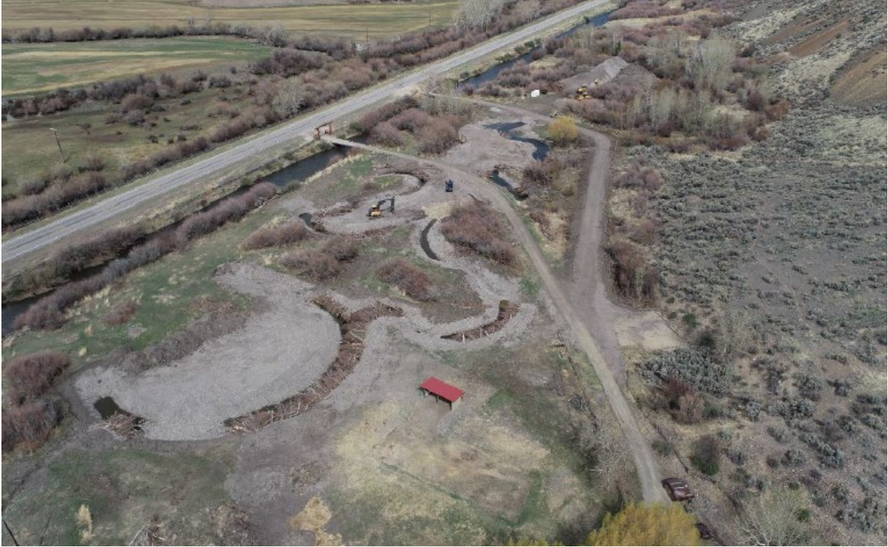
Figure 18: 2023068: Downstream of Project
