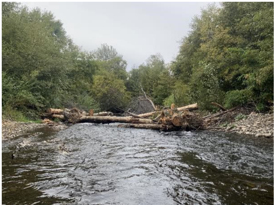
Figure 2: 2023004(Tucannon PA-26) LW Structure2
