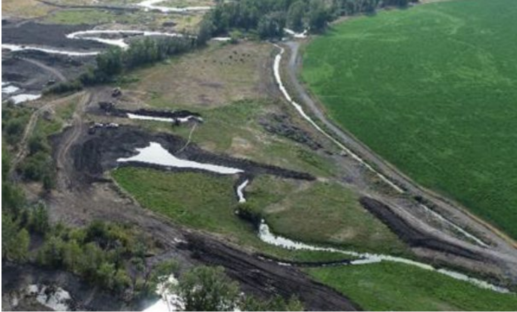
Figure 19:2023070: Construction of Idaho Complex and relic beaver dams
