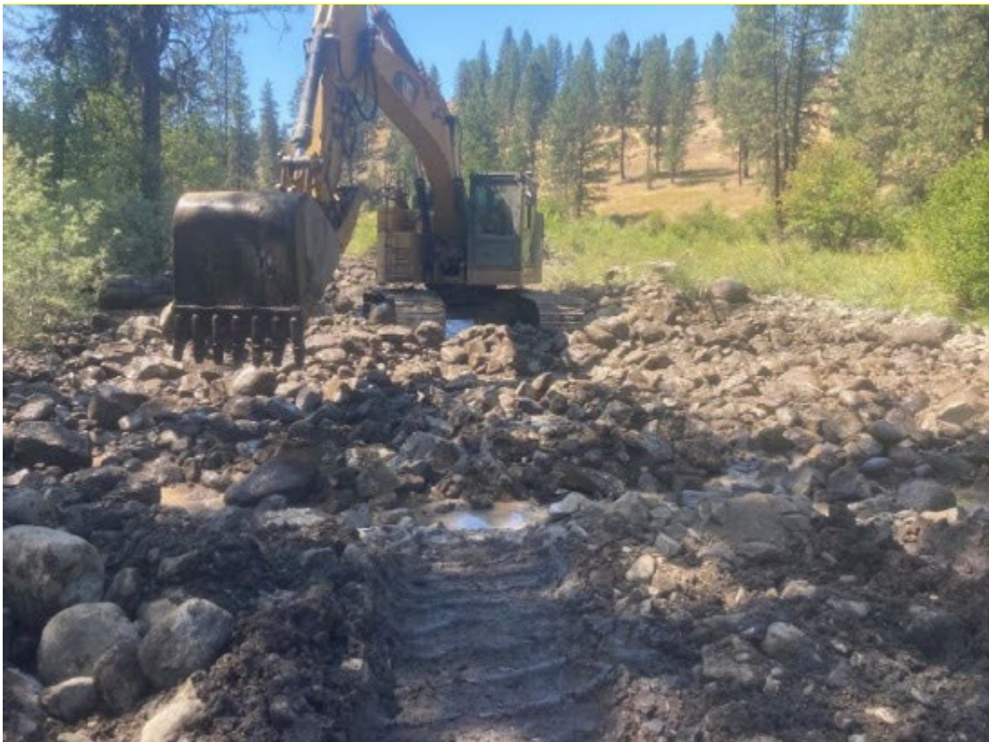
Figure 26: 2023072(Desolation Creek)Riffle_Construction
