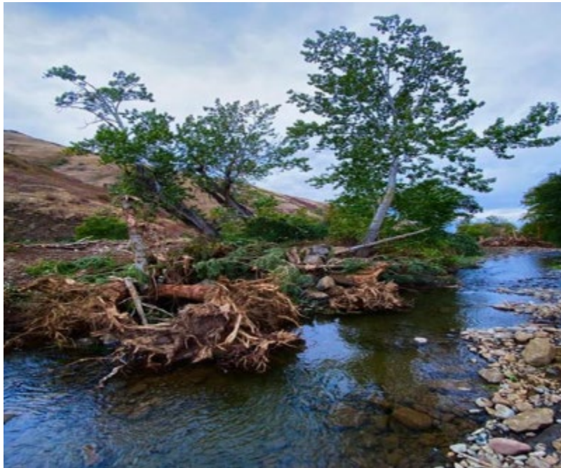
Figure 29: 2023074: Post Construction root wads into created pools
