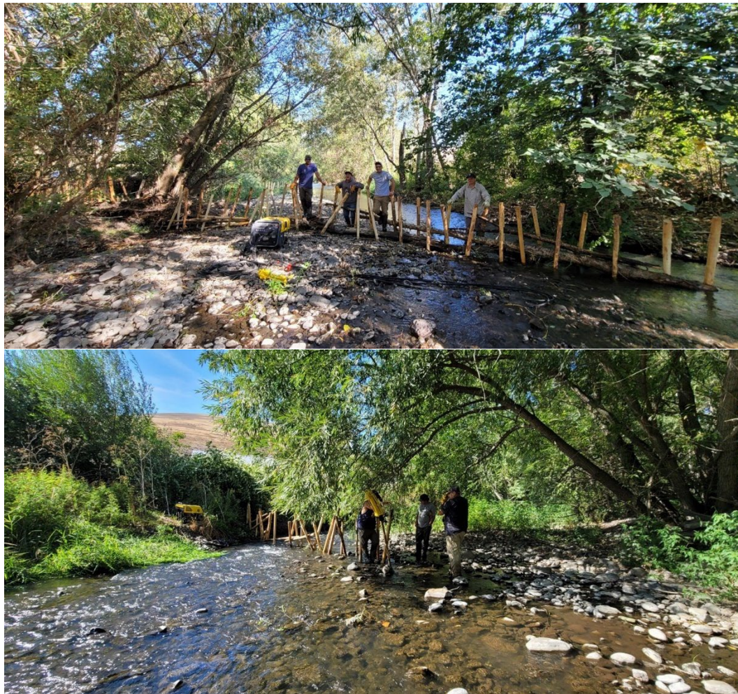
Figure 3: 2023088(Lapwai Creek)BDA Install
