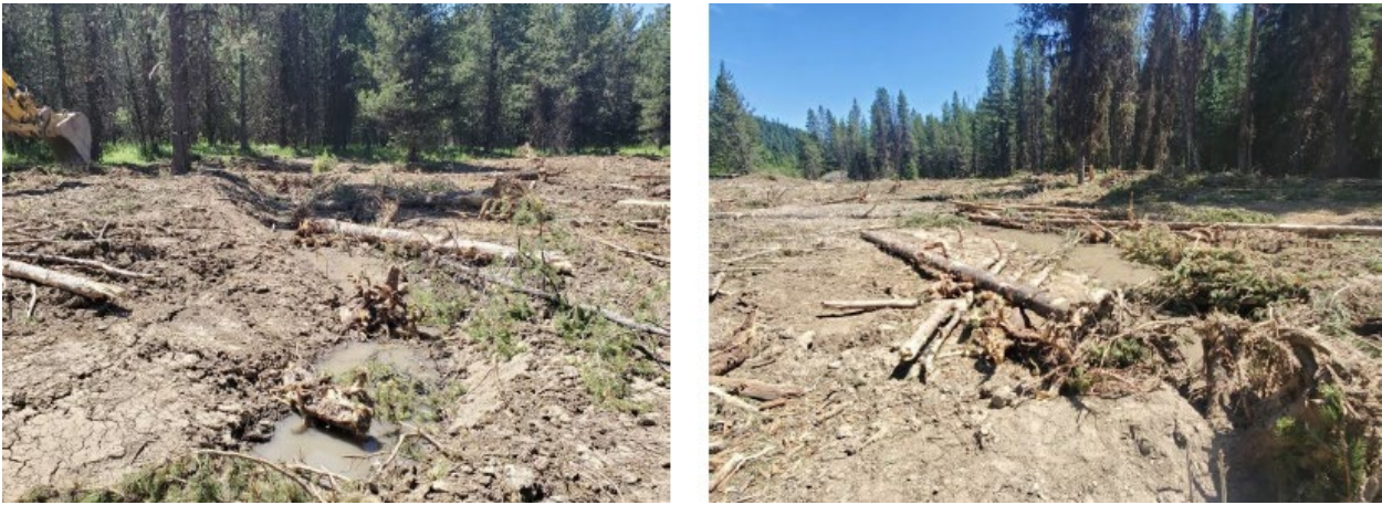
Figure 9: (2023008) Excavated Channel after wood installation
