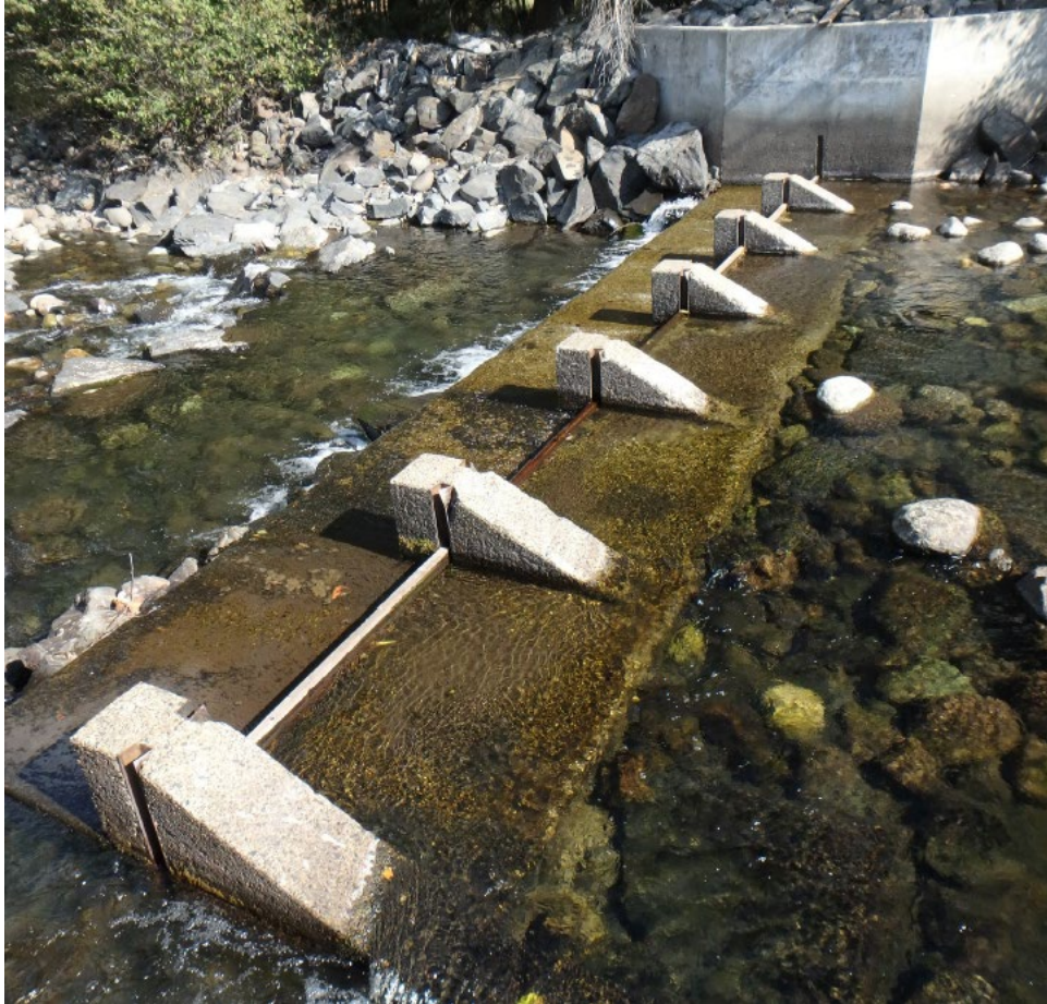
Figure 13: 2023009: Lowered weir
