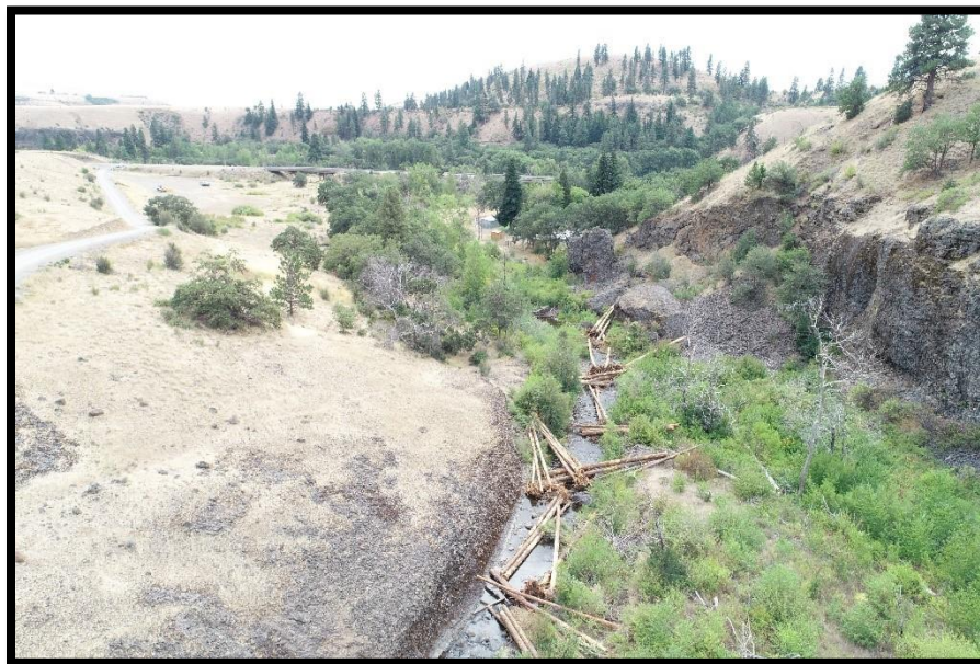
2019091(YKFP) Large Wood Placement
