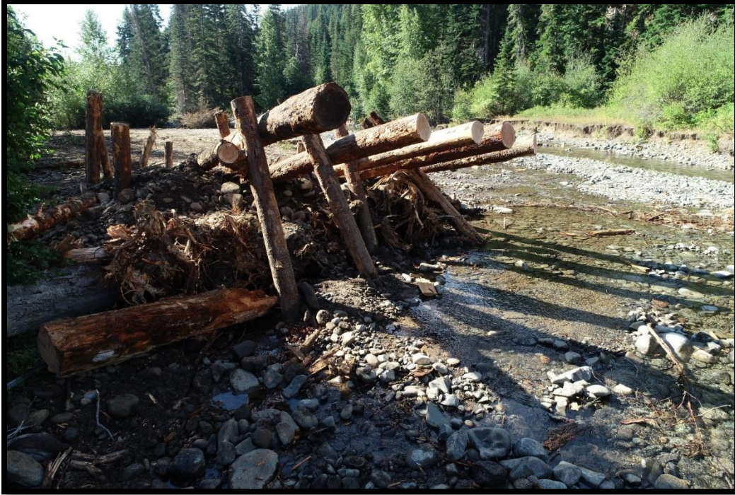
2019093 (North Fork Teanaway) Large Wood Jam.
