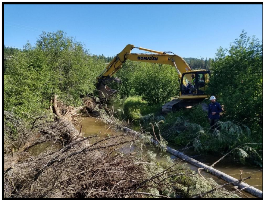
2019052(Dammerman) Large Wood Placement
