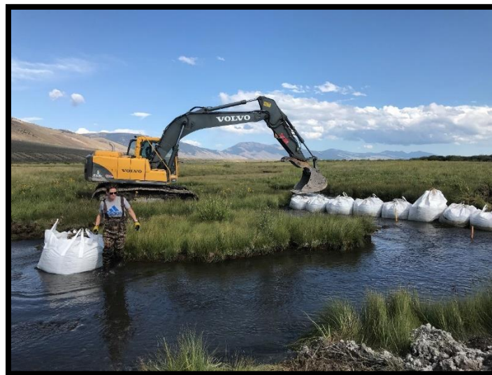
2019076 (L-61) Cofferdam Installation
