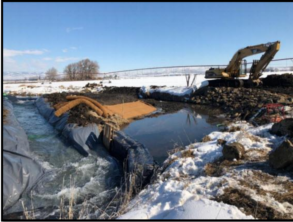
2019013(Caribou Creek) After removal, note bare earth
