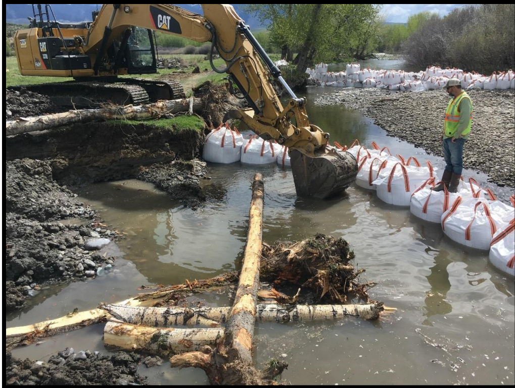
2019050 (Lehmi River Restoration) Cofferdam and large wood placement
