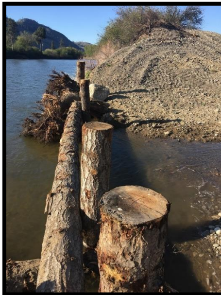
2019108(Pharr Road)Large Wood Placement
