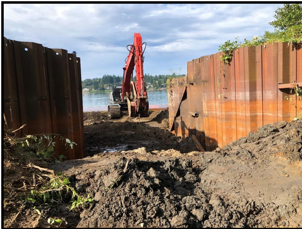
2019071 (Govt Island) Levee Removal
