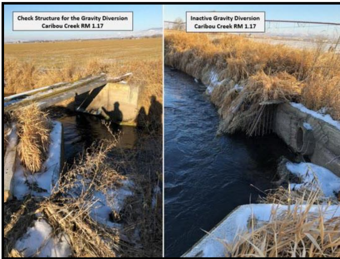
2019013(Caribou Creek) Structures before removal
