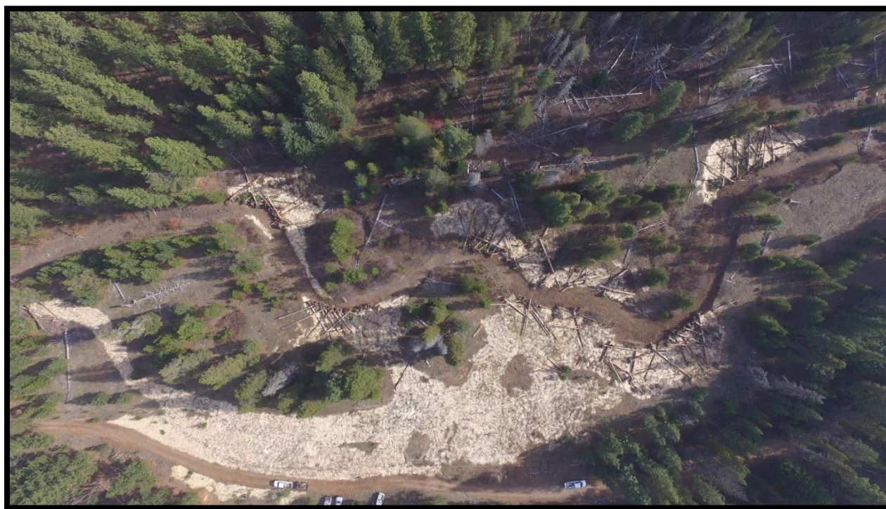
2019053 (White Creek) Channel Reconstruction
