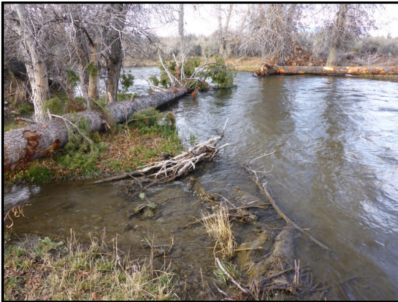
2016072: Pahsimeroi Floodplain Restoration
