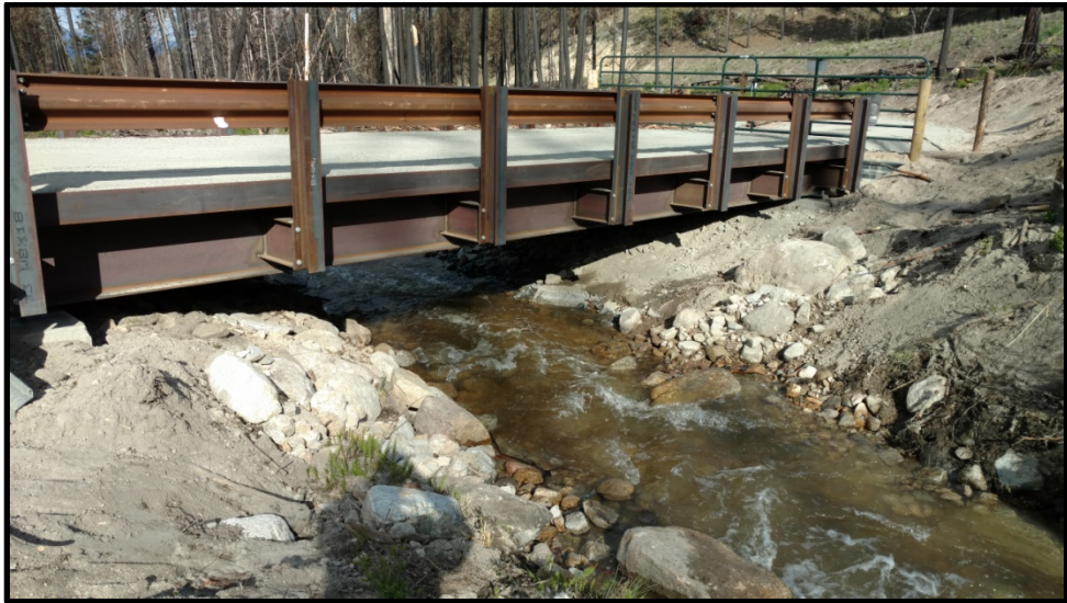
2016012: Parker Bridge Replacement (After)
