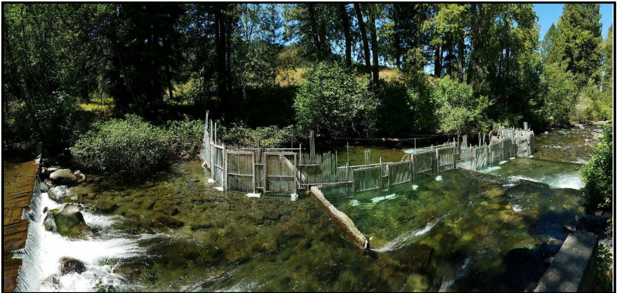
2016033: Lostine Diversion Removal – Exclusion Barrier.
