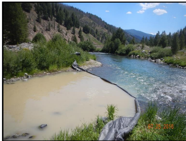
2016009: Photos show work area isolation measures are competent and effective.
