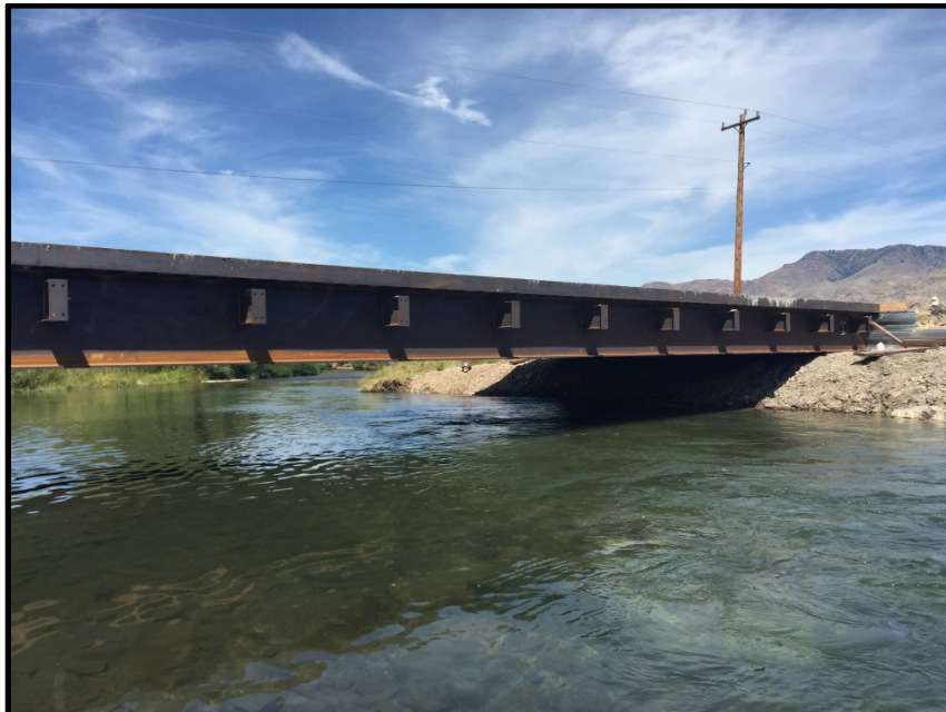
2016031: Downtown Lane Culvert Replacement (After).
