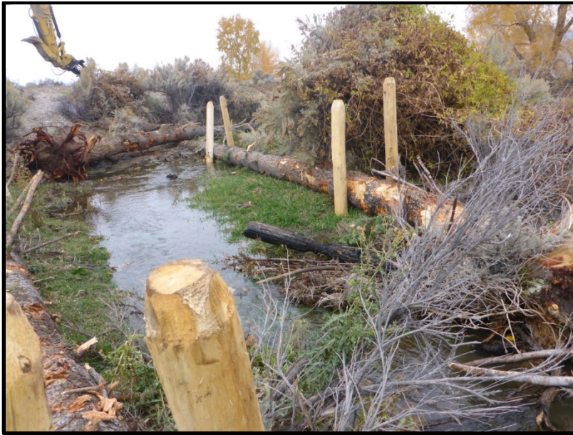
2016072: Pahsimeroi Floodplain Restoration
