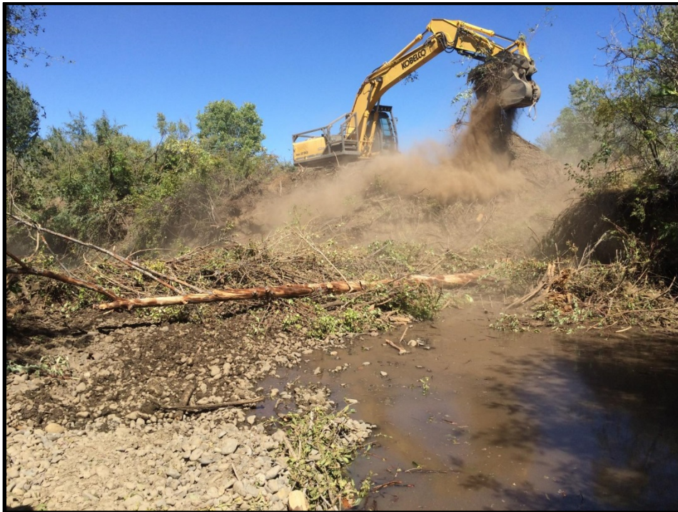
2016039: Toppenish Bank Restoration.
