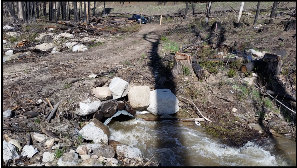
2016012: Parker Bridge Replacement (Before)
