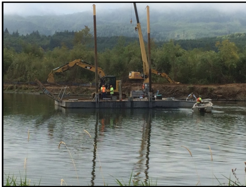
2016033: Westport Slough Levee Removal
