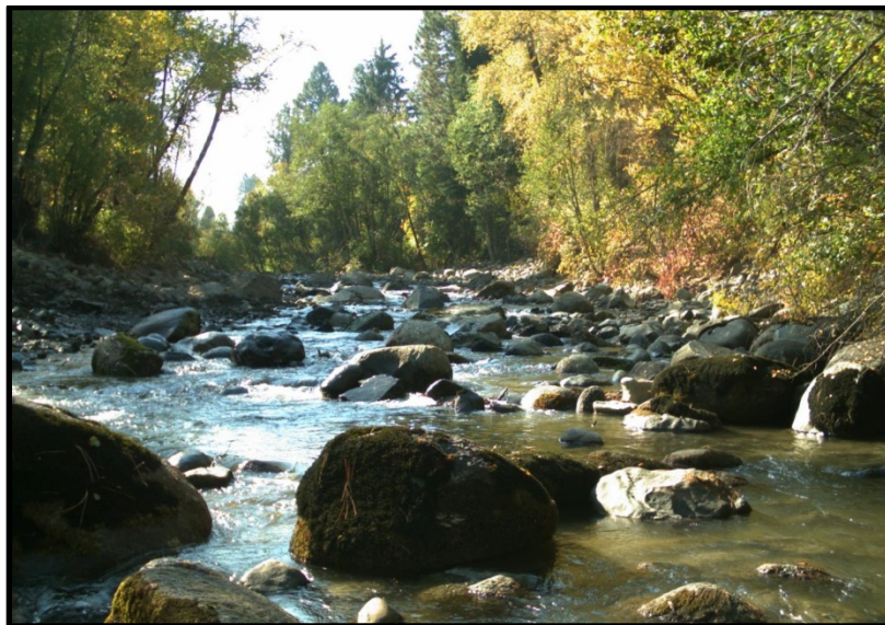
2016033: Lostine Diversion Removal (After)
