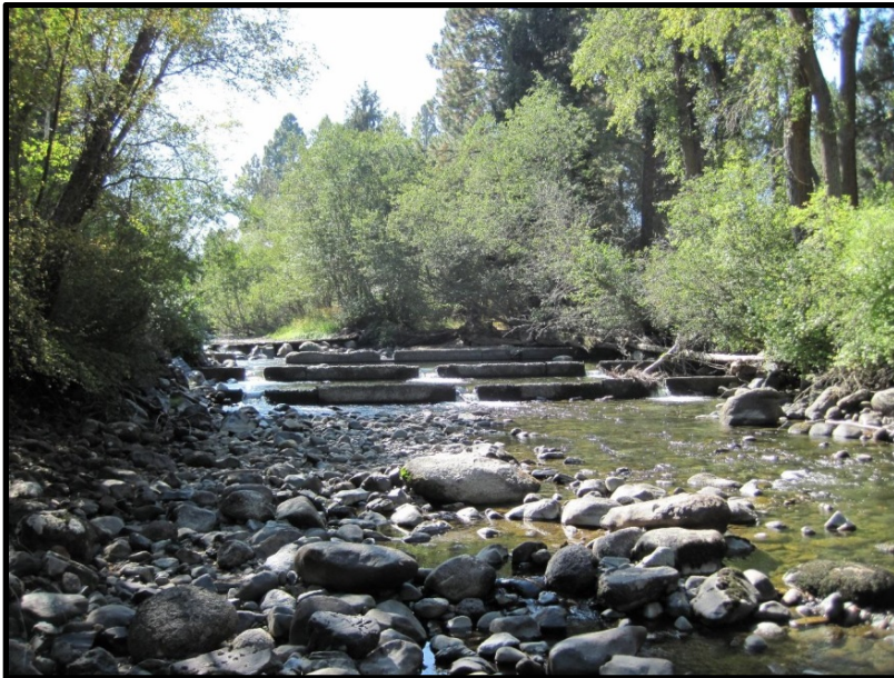
2016033: Lostine Diversion Removal (Before)
