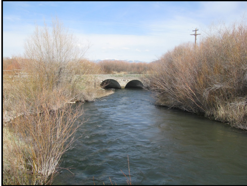
2016031: Downtown Lane Culvert Replacement (Before).
