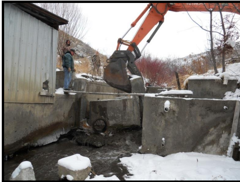
201442 Antoine Creek Diversion Removal (Before)
