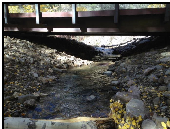
201499 Bayhorse Creek Culvert to Bridge Replacement (After)
