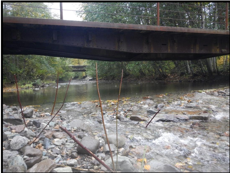
201498 Big Creek Fish Passage Project (After)
