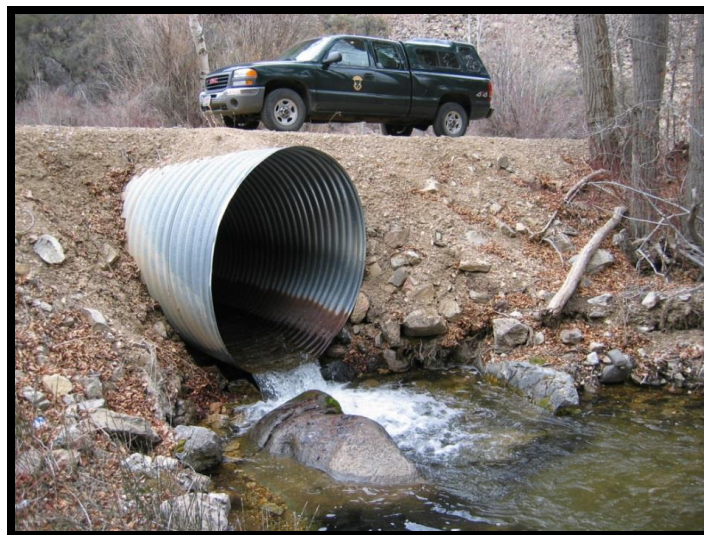
201499 Bayhorse Creek Culvert to Bridge Replacement (Before)
