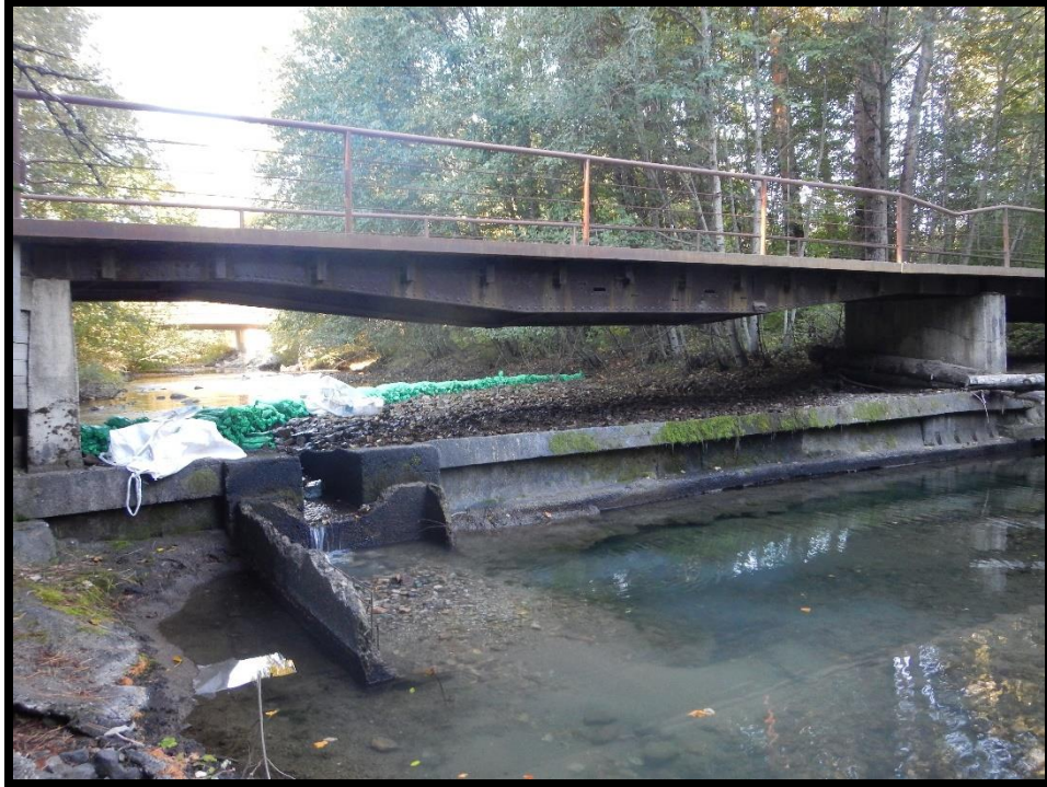
201498 Big Creek Fish Passage Project (Before)
