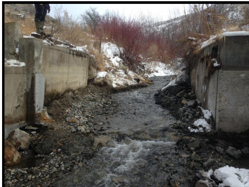
201442 Antoine Creek Diversion Removal (After)
