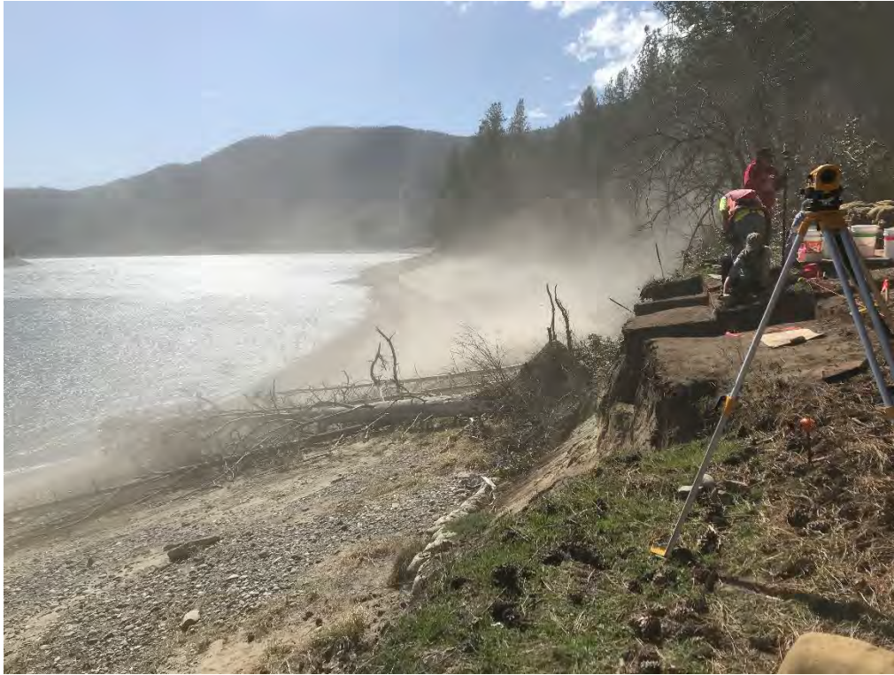
Figure J-6. CCT H/A staff excavating an eroding bank at 45ST1111.
