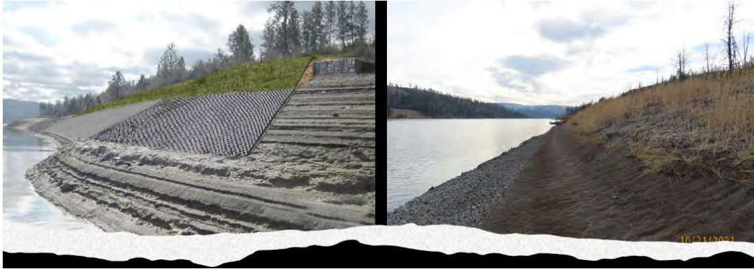
Figure J-4. Comparison of artist's concept (left) 45LI377 stabilization to the actual implementation (right) shows that the stabilization appears as hoped. Note that "manta ray" anchors are used instead of the more expensive and impactful gabion baskets.
