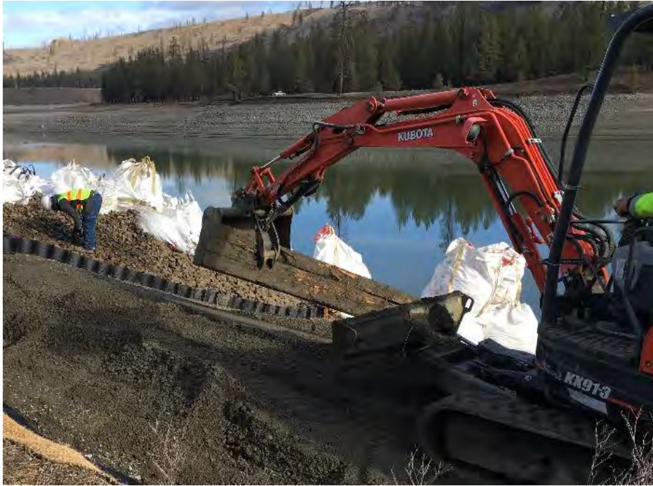
Figure J-2. Site stabilization construction at site 45LI377.
