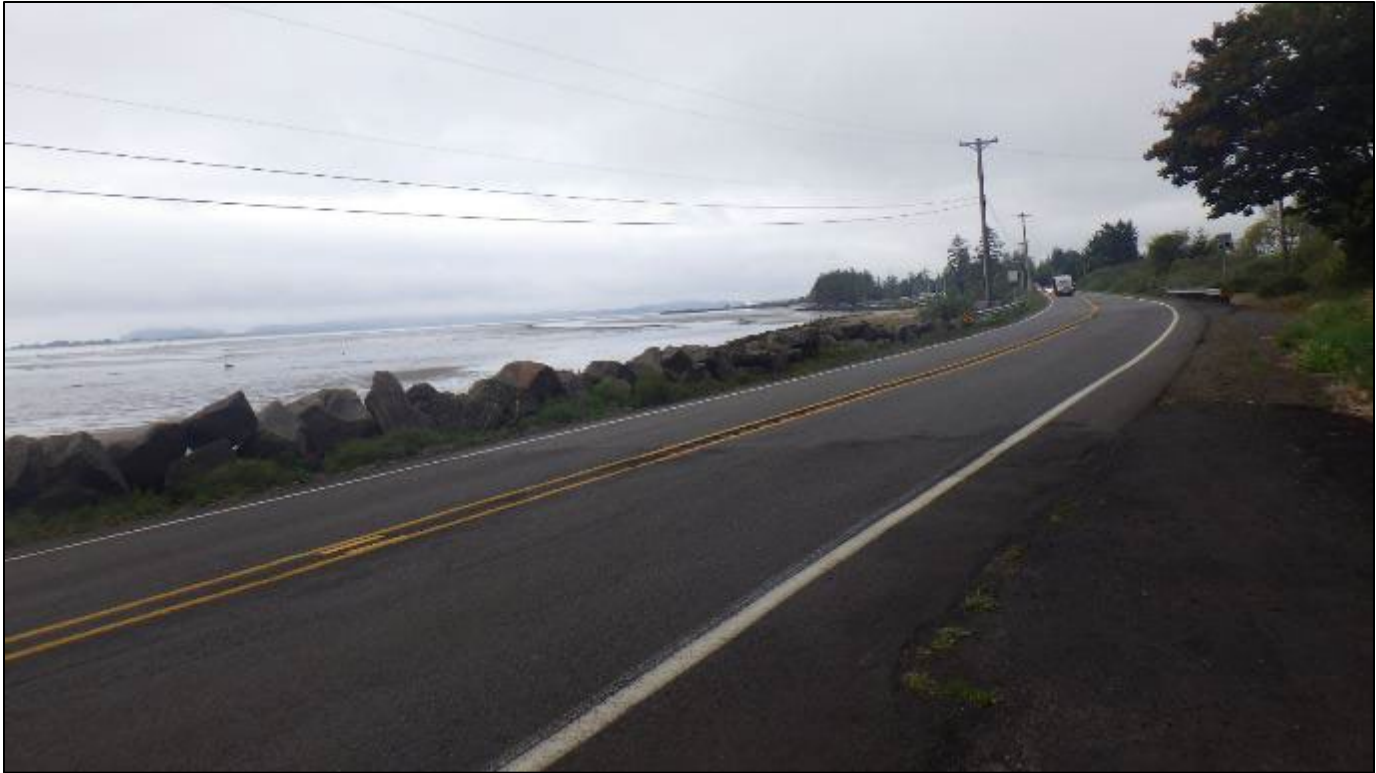
Photo 1. U.S. 101, a federal levee along the Columbia River in Pacific County, view north, 2025, HRA.
