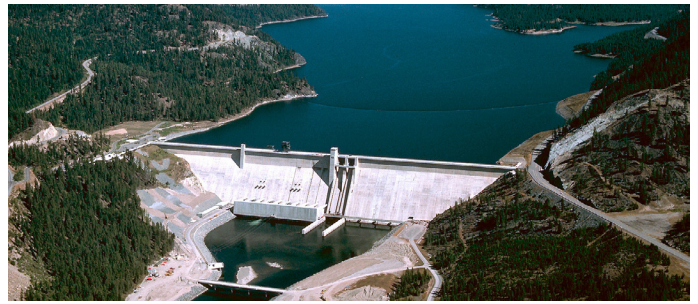
Libby Dam spans the Kootenai River 17 miles upstream from the town of Libby, Montana. The Kootenai River is the third largest tributary to the Columbia River, contributing almost 20% of the total water in the lower Columbia River. The dam began operating in 1975, forming Lake Koocanusa, and is owned and operated by the U.S. Army Corps of Engineers, Seattle District. Acting partially as a storage reservoir, Lake Koocanusa extends 90 miles upriver from the dam and has a maximum depth of about 370 feet. Constructed under the Columbia River Treaty, 48 miles of the reservoir lie within the borders of the U.S.; the remaining 42 miles are in Canada. The reservoir name, Koocanusa, is the combination of letters from the Kootenai River, Canada, and the U.S. lands surrounding the reservoir. Cultural resources present there continue to provide physical connections to traditional practices and beliefs of the Confederated Salish and Kootenai Tribes.
