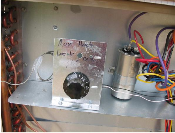
Ohmmeter between the control terminals, and turn the adjustment dial until the circuit is closed (resistance on ohmmeter goes from infinite to 0 or near 0). If the circuitry does not make/break right around 32° F, the control will have to be exchanged for another control.
