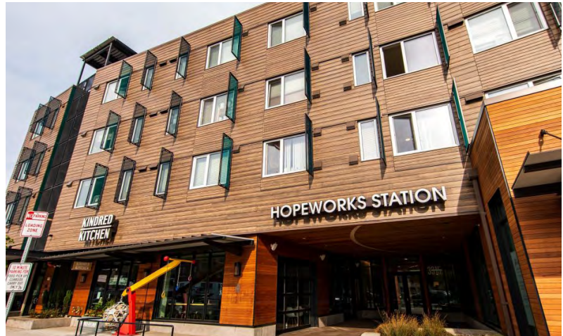
Hopeworks Station in Everett, Washington.
