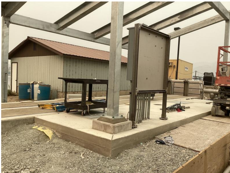
New UV System in Construction
