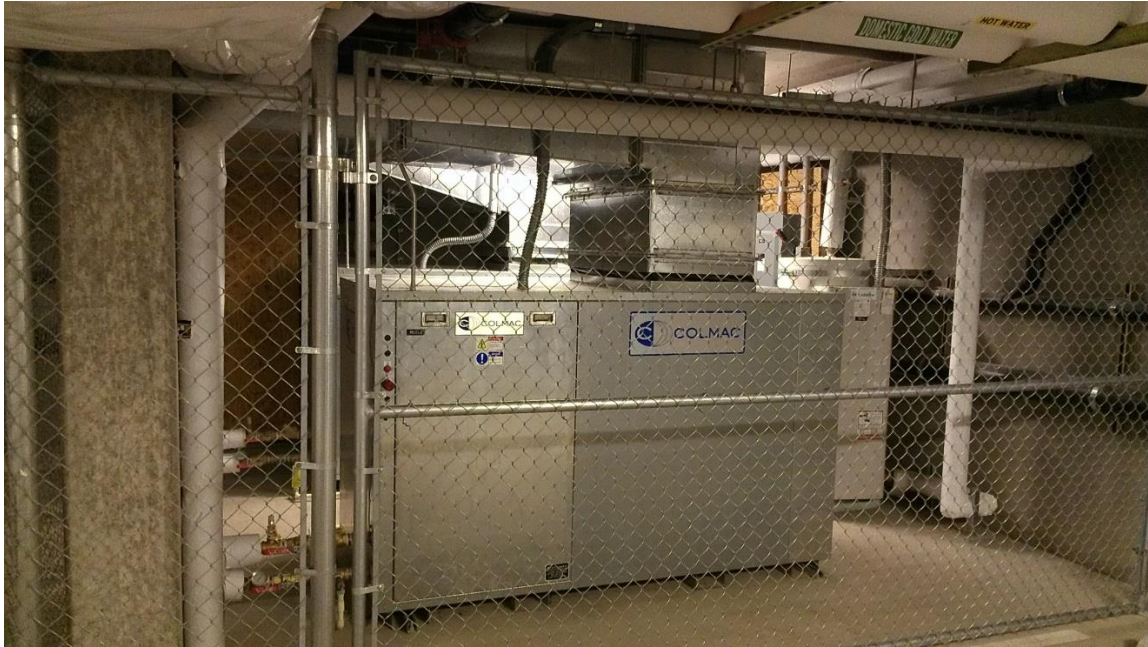
Photo 1: RCC's Looking West
