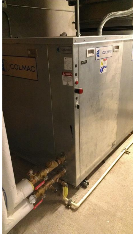
Photo 3 & 4: RCC Discharge Location and RCC Piping Connection
