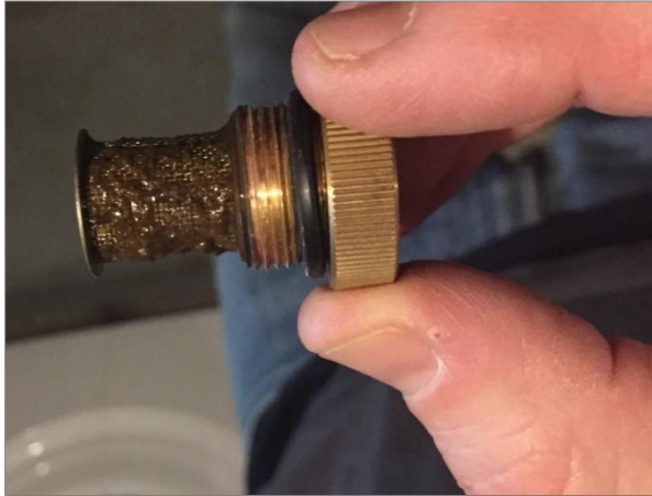
Figure 19. Clogged Filter at Portland Site
