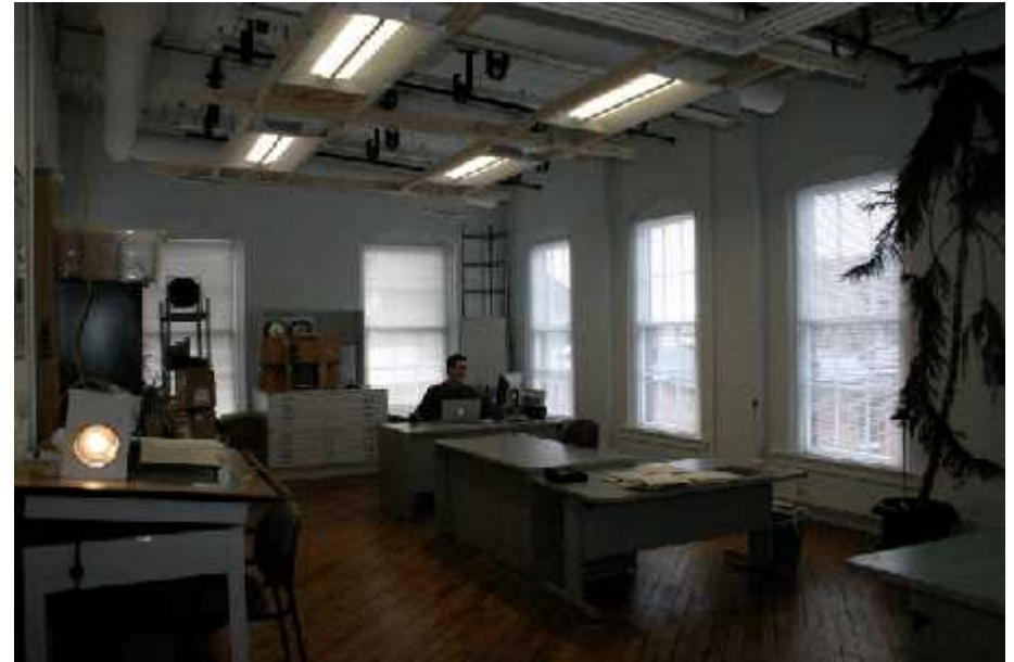
Open office space with Cree LED luminaires
