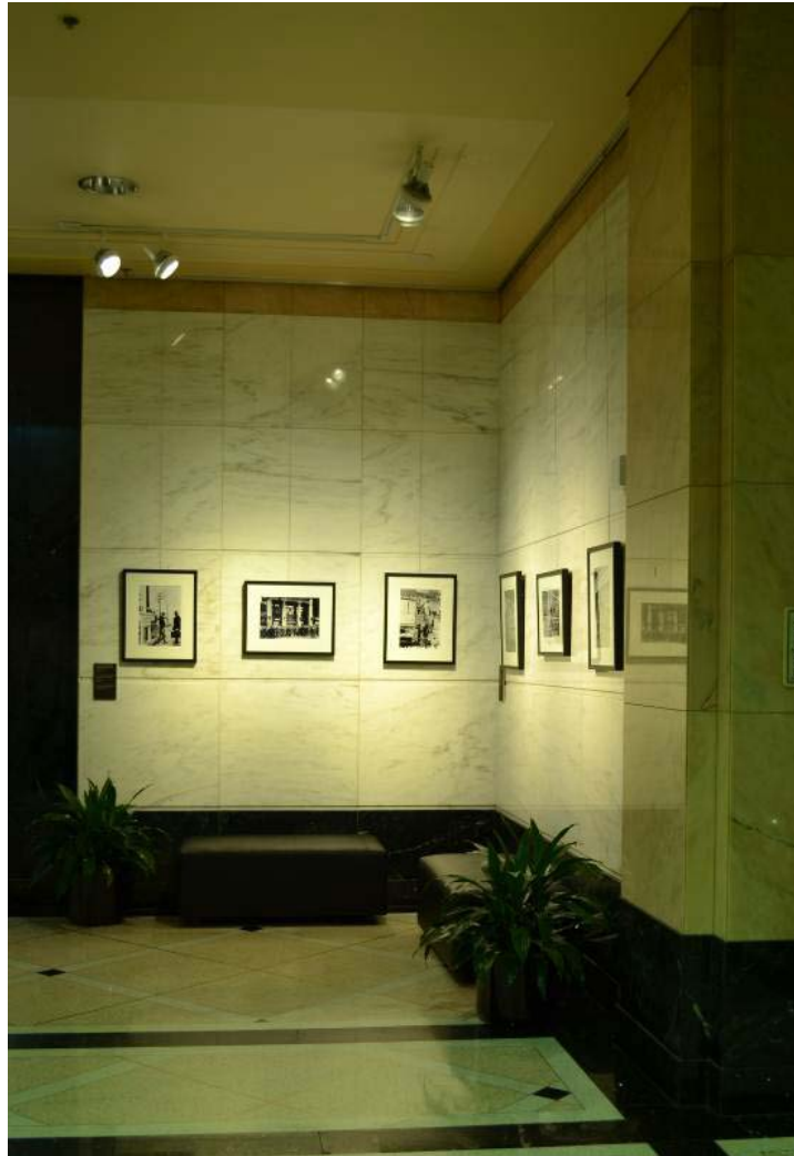
Figure 4. Lobby photos lighted with Cree LRP38 LED lamps (AFTER). Note that the beam is much more focused on the intended target. (Photo by Mike Hoffman, PNNL.)
