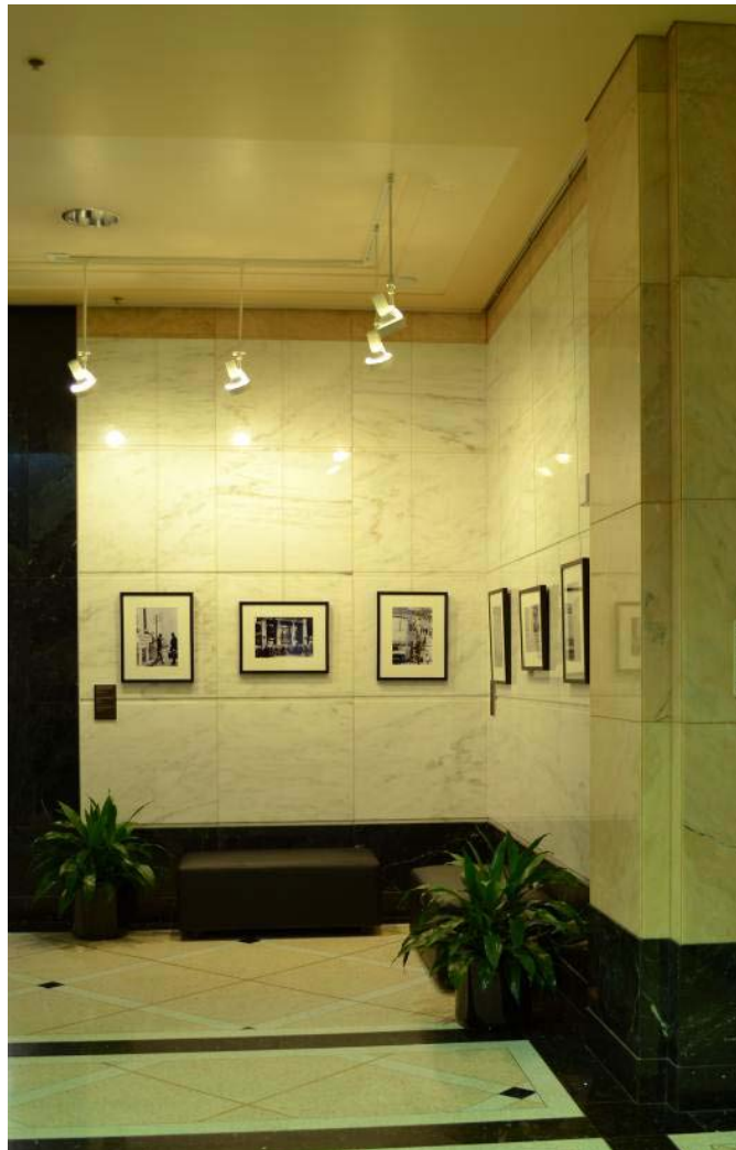
Figure 3. Lobby photos lighted with Philips EL/A R30 compact fluorescent lamps (BEFORE). Note high level of illumination above the artwork. (Photo by Mike Hoffman, PNNL.)
