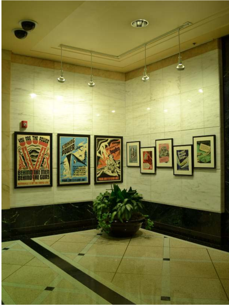
Figure 5. Lobby poster art lighted with TCP FP3823 PAR38 compact fluorescent lamps (BEFORE). (Photo by Mike Hoffman, PNNL.)
