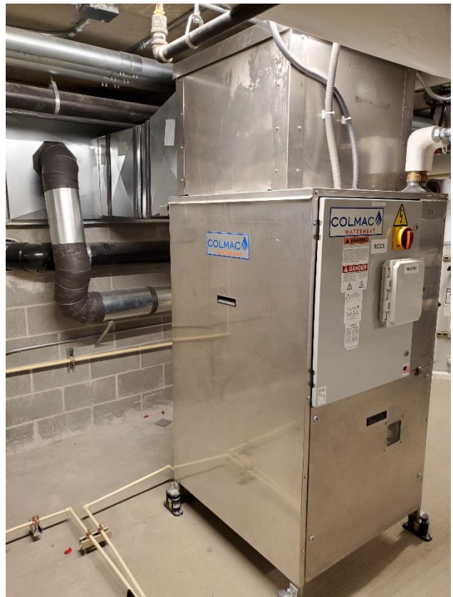
Figure 4. HPWH-5, one of two primary CxA HPWHs
