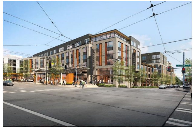
Figure 2. Jackson Apartments in Seattle, WA (Source: Apartments.com)
