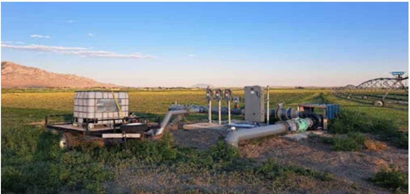
Inskip pipeline farmer tie-in.
