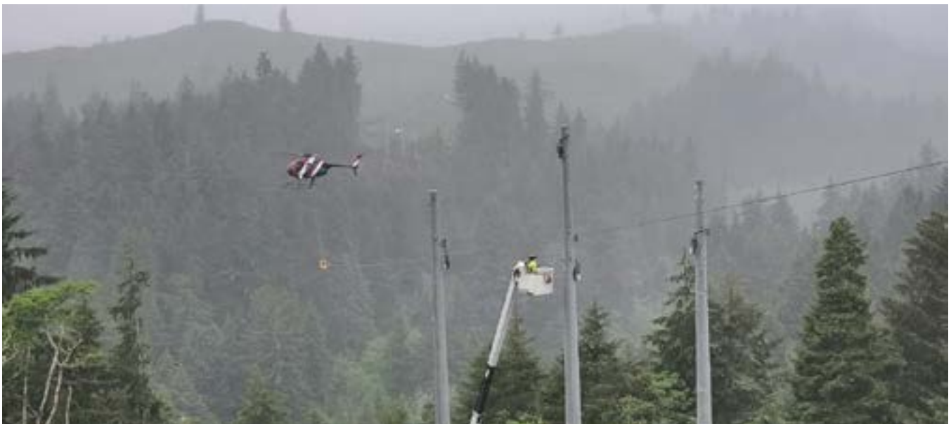
A helicopter guides conductor during the installation of Central Lincoln PUD's new 69-kilovolt transmission line leading to Newport, Oregon. The pole structures stand 115 feet tall.
