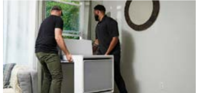
Saddle style packaged window heat pump.
