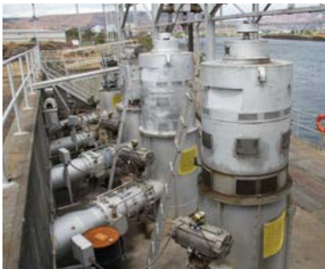
Dalles Irrigation District River Station pump upgrades.
