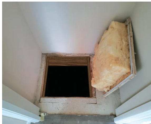
Indoor access door/hatch for underfloor areas: Weatherstrip and securely insulate all inside access doors. Image courtesy of Dan Wildenhaus
