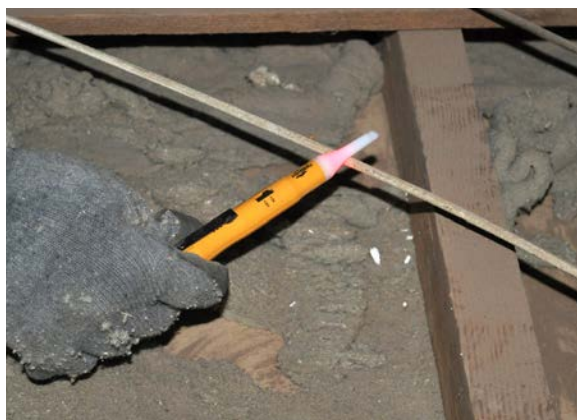
Non contact voltage tester: Test voltage wires near your work area and turn off the circuit if appropriate. Image courtesy of Energy Smart Academy
