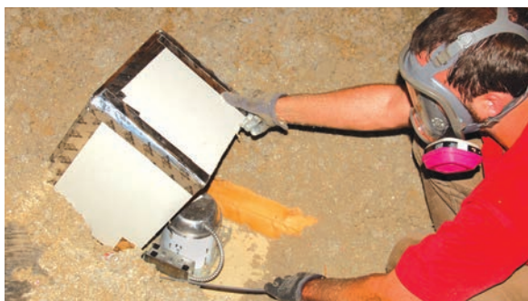
Air-sealed drywall box: This airtight drywall box serves as both an air seal and an insulation shield. Image courtesy of Energy Smart Academy
