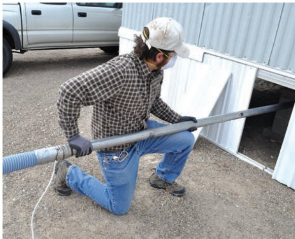
Blowing through rodent barriers: A flexible fill-tube, which is significantly stiffer than the blower hose, blows fiberglass insulation through a hole in the belly from underneath the home. Image courtesy of Energy Smart Academy
