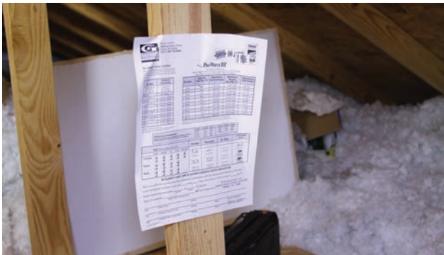
This is an example of an Installer Record permanently posted at the electrical panel or other location approved by homeowner. Installers are responsible for the creation of their own Installer Record.
