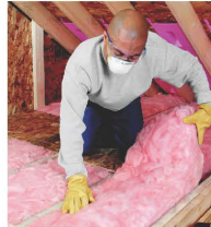
Batt Insulation Installation
