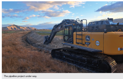
The pipeline project under way.
