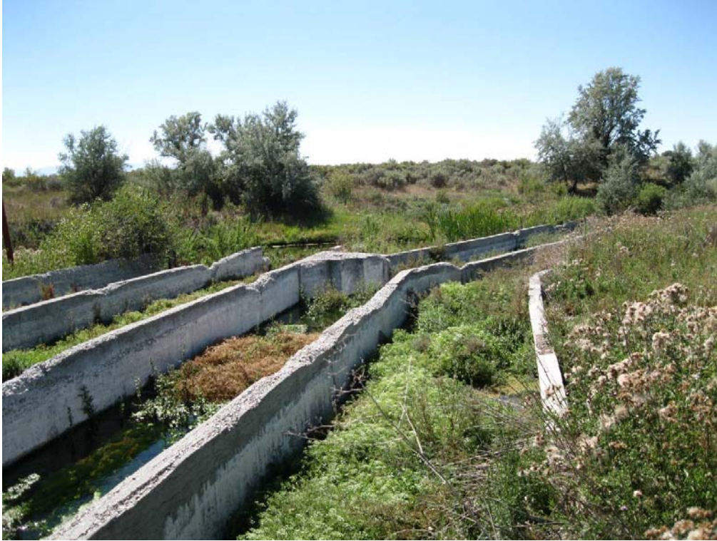
Figure 4-6. Abandoned raceways at the Crystal Springs Hatchery site.
