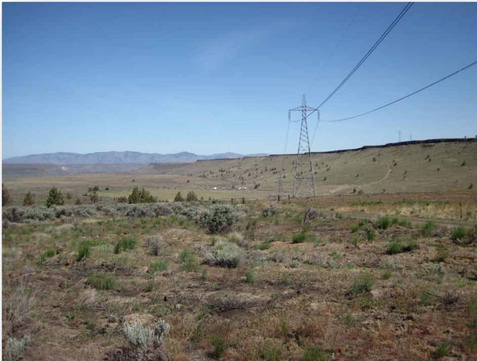
Figure 3.9-2: Transmission Line Crossing of US 97 at Tower 61/1
