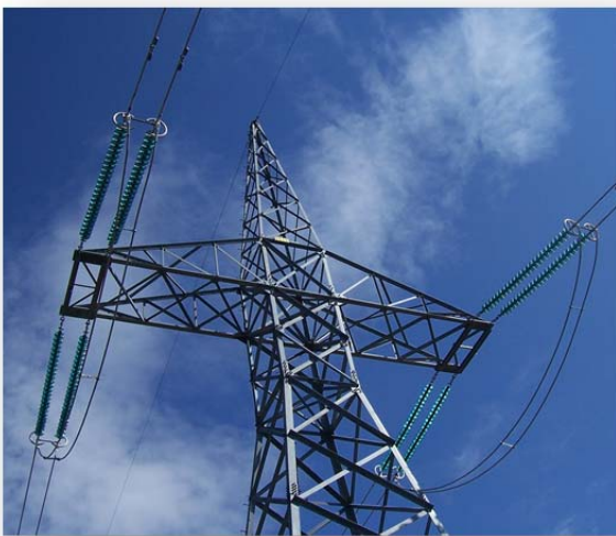
Figure 2.1-7: Glass Insulators on Dead-end and Rigid Insulators on Guyed Tower
