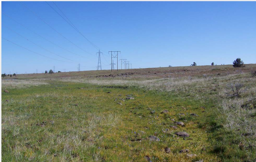
Figure 2.1-3: Existing PDCI Line North of US 97-US 197 Intersection (looking north from Tower 48/1, Big Eddy-Redmond No 1 is on the right)
