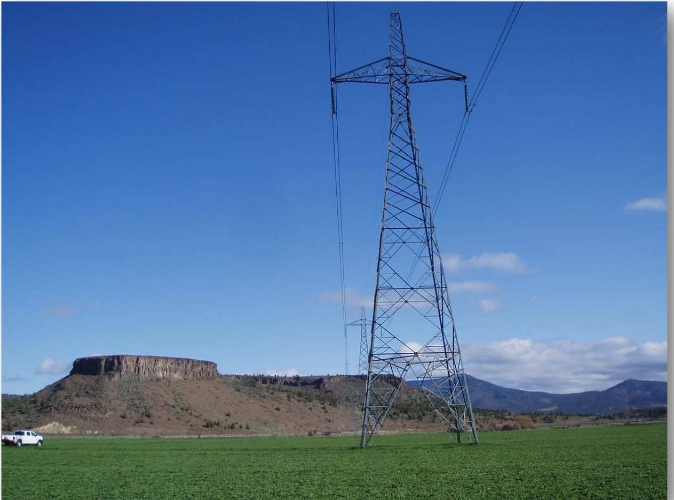
Figure 2.1-3: Existing PDCI Line Irrigated Agricultural Land South of the Crooked River (Tower 91/2 looking south)
