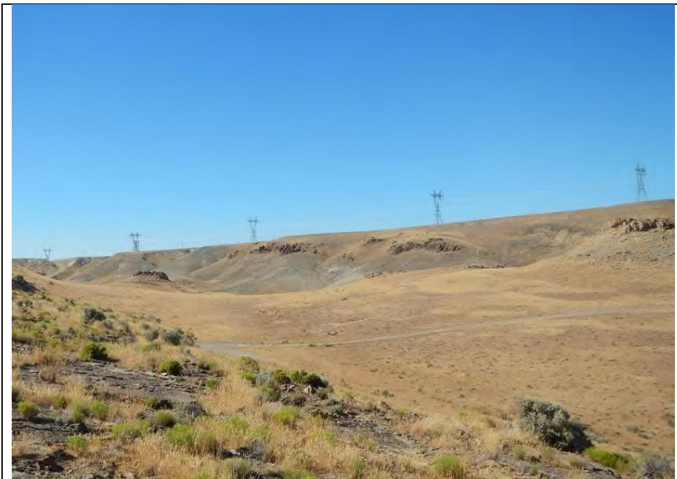
Figure 3-1. Example of Visibility Conditions
