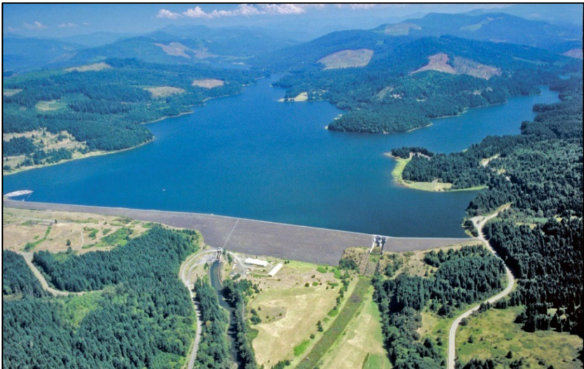
Figure 4-5. Fall Creek Dam and Reservoir.
