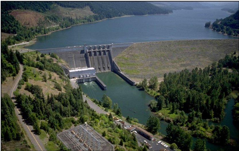
Figure 4-3. Lookout Point Dam and Reservoir.
