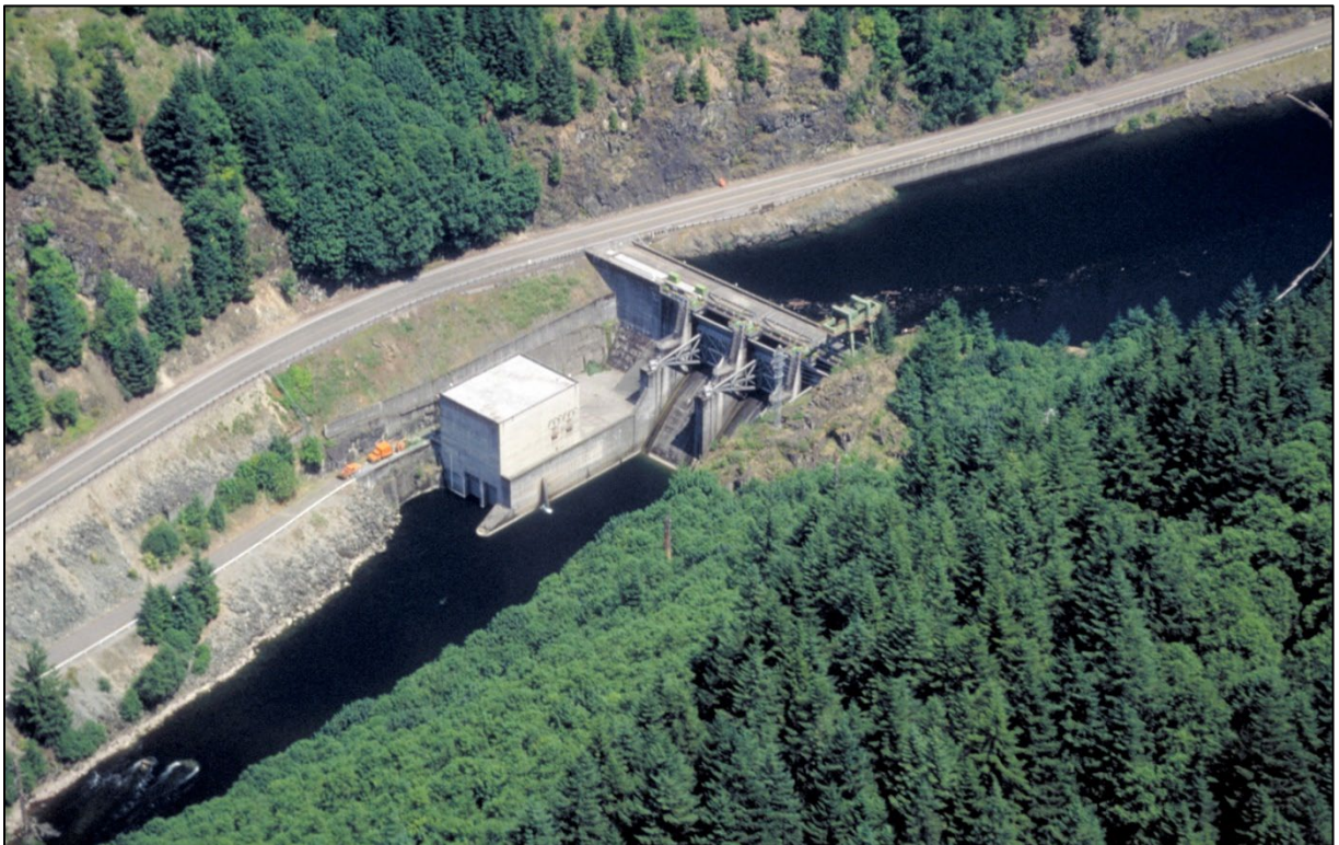
Figure 4-19. Big Cliff Dam and Reservoir.
