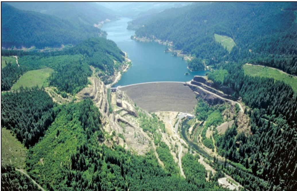
Figure 4-11. Cougar Dam and Reservoir.
