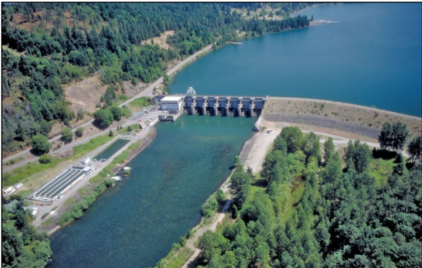
Figure 4-4. Dexter Dam and Reservoir.
