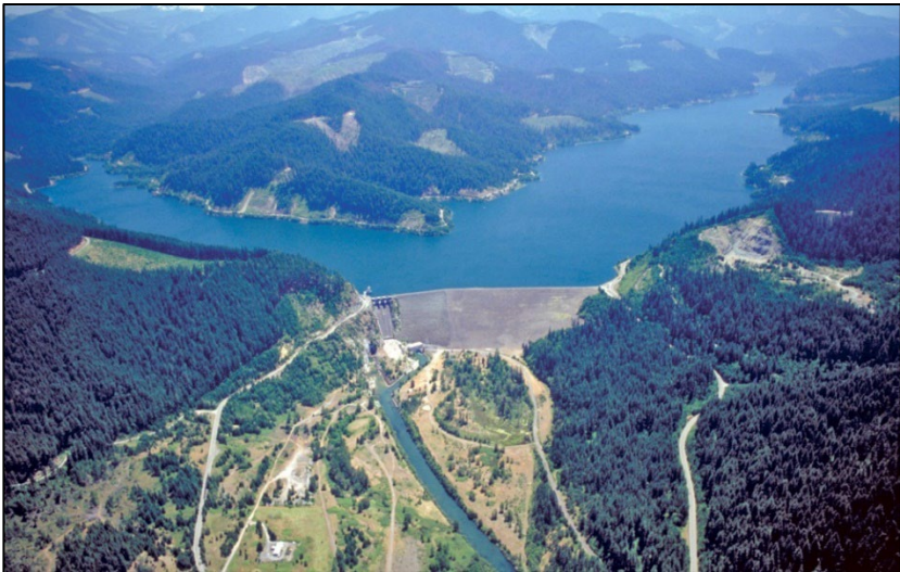
Figure 4-2. Hills Creek Dam and Reservoir.
