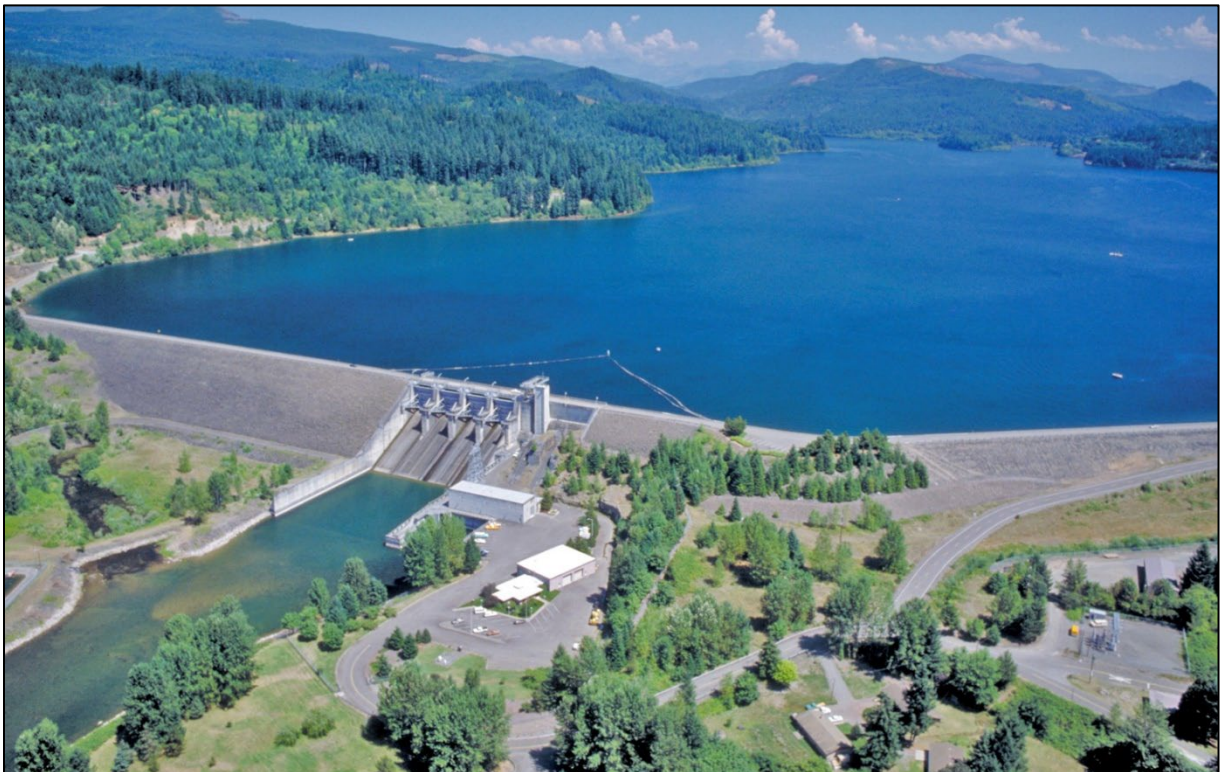
Figure 4-16. Foster Dam and Reservoir.
