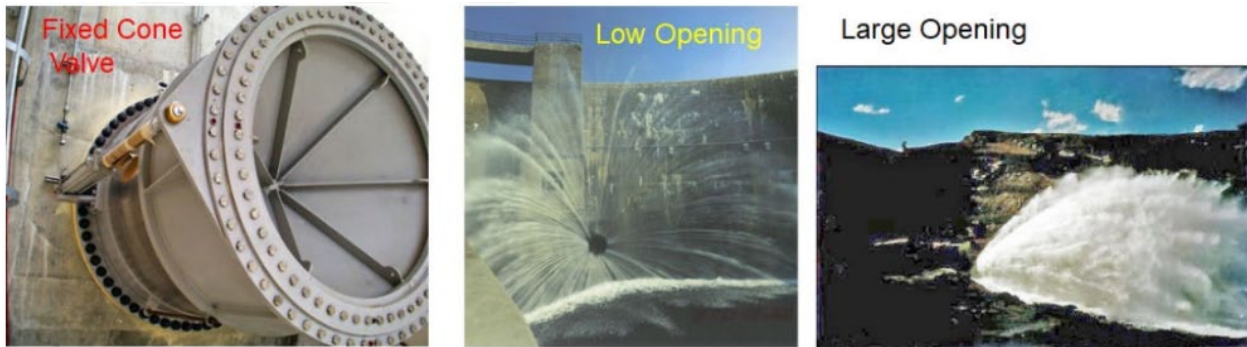
Figure 1-1 Standard Cone Valve with Conical Spray at Boulder Dam, Colorado.
