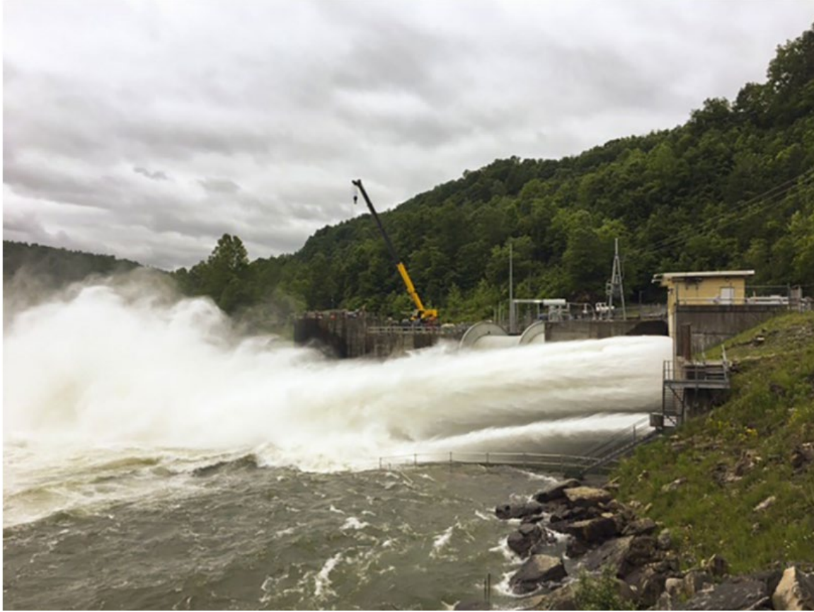
Figure 1-2 Hooded Cone Valve Operations at Summersville Dam, West Virginia
