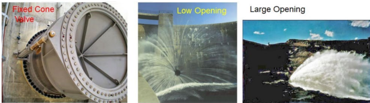
Figure.7.7.Standard.Cone.Valve.with.Conical.Spray.at.Boulder.Dam?Colorado;
