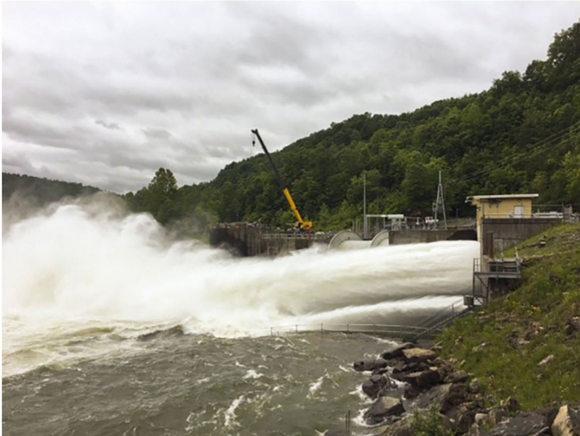
Figure.7_8.Hooded.Cone.Valve.Operations.at.Summersville.Dam?West.Virginia
