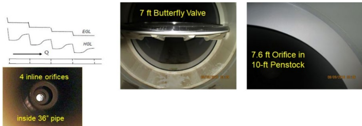
Figure.7_9.In_line.Orifice.Systems.inside.Pipelines.(Seven.Oaks.Dam?lower.left?.The.Dalles.Dam?upper.middle.and.right)
