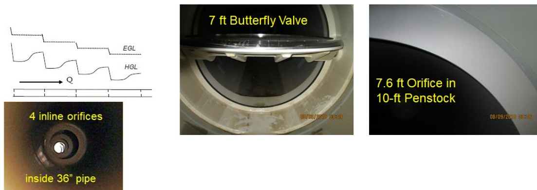
Figure 2-14. In-line Orifice Systems inside Pipelines (Seven Oaks Dam, lower left; The Dalles Dam, upper middle and right)
