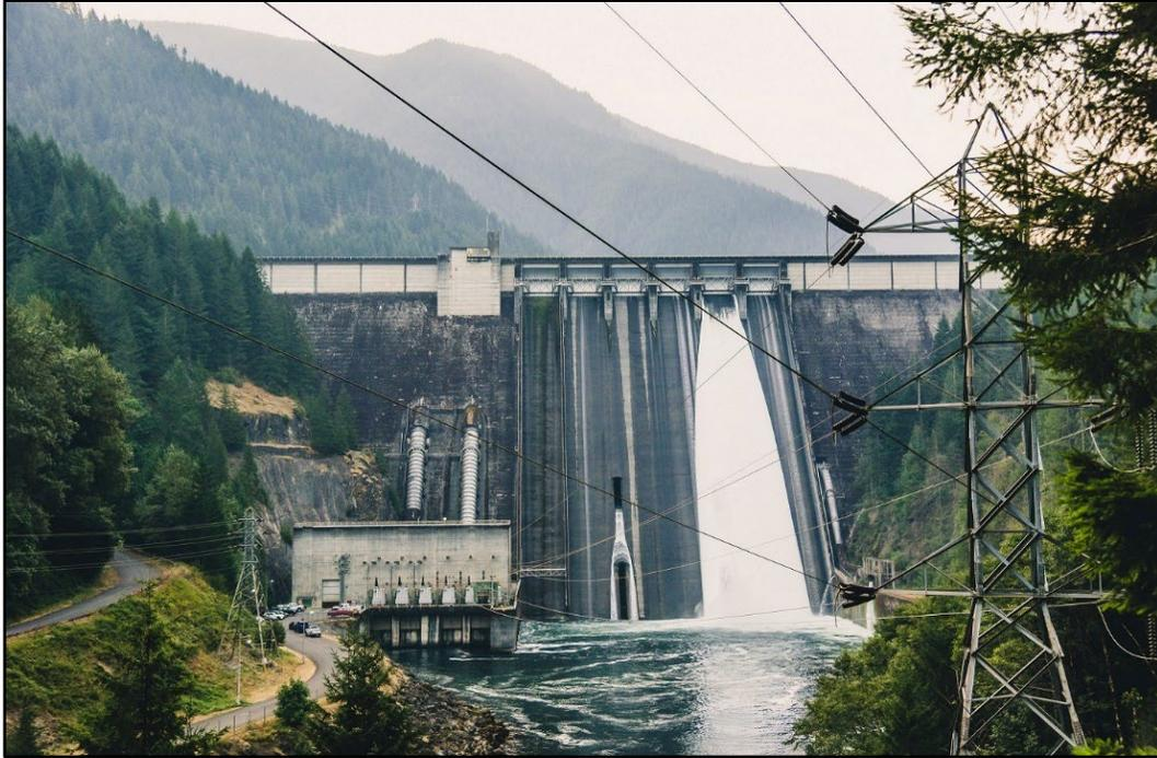
**Figure 1.10-3. Transmission Lines Extending from the Powerhouse at Detroit Dam.**
