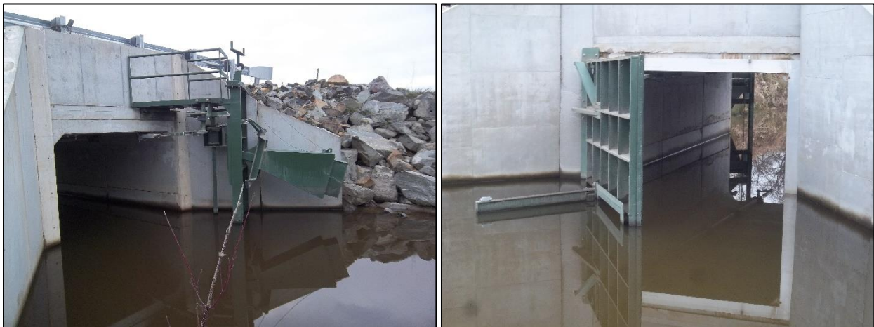
Figure 2-2: Example concrete box culvert with automated tide gate proposed for the Auto Tour Route and Deep Creek Breach.
