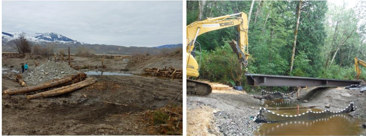
Figure 4 Large-scale vs small-scale impacts from construction activities on restoration projects
