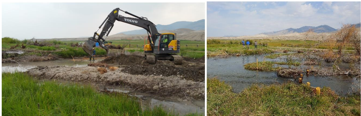
Figure 9 Example of degree of disruption during and after stream restoration action in same year
