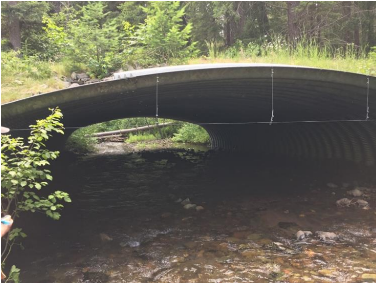
Figure 4 Photo of an example open bottom arch culvert that would replace the undersized culvert at the Whiskey Creek Road crossing.
