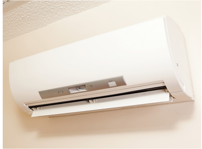
A wall-mount mini-split heating and air conditioning unit.
